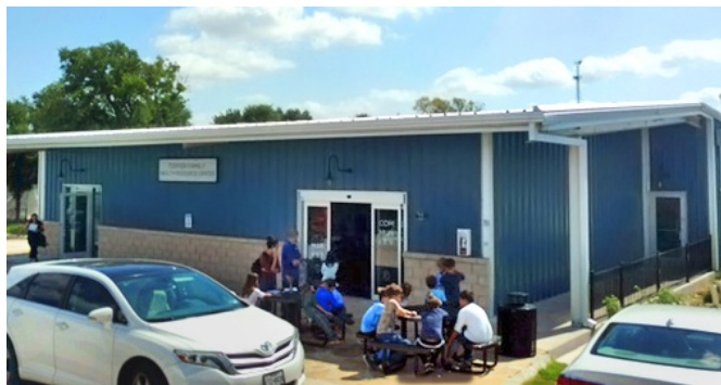
Community First! Village's services building featuring bath and laundry facilities, as well as the village's medical clinic.
